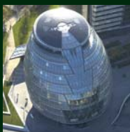
Photovoltaic energy generation: Foster + Partners' City Hall, London 太陽板發電 Foster + Partners 設計的倫敦大會堂
